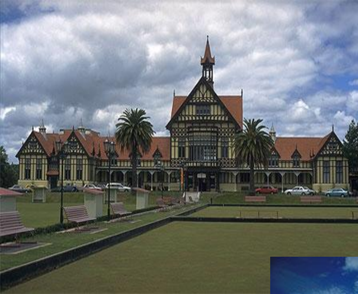
The Tudor towers of Rotorua's Bath-House
