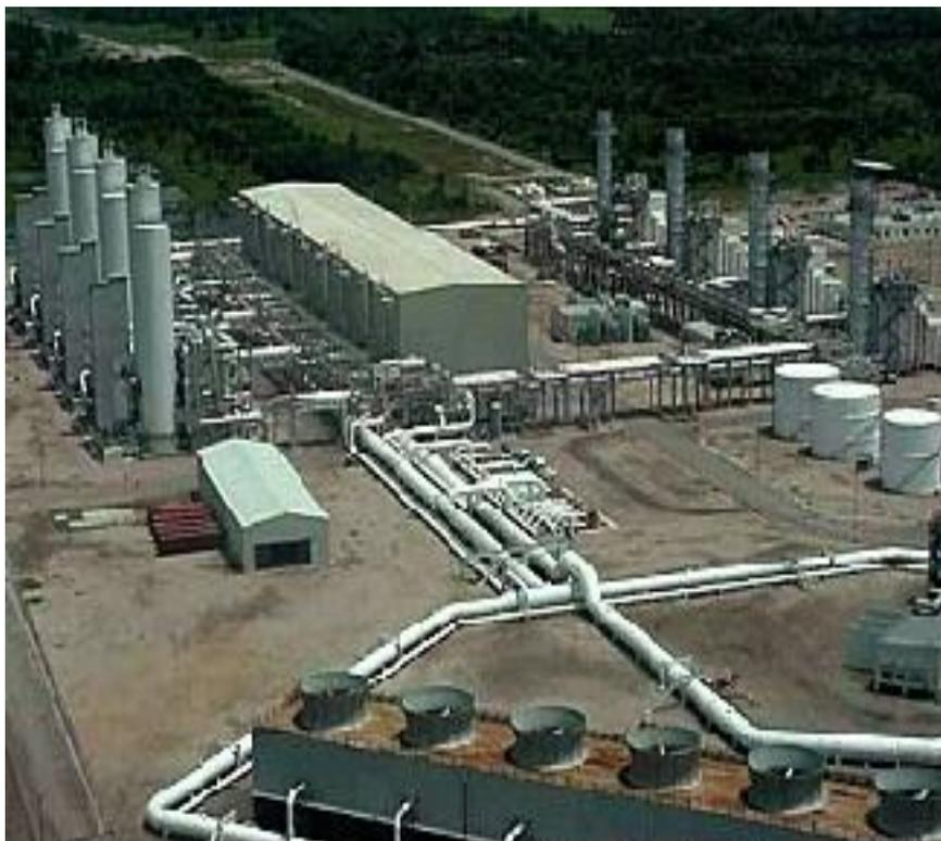
The four nitrogen-production units stand at the right in this view of the Cantarell nitrogen-generation plant. The compression housing is in the middle, the four power-generation units are to the right with water coolers shown at the bottom (Fig. 1). Photograph from Compañía de Nitrógeno de Cantarell and Petróleos Mexicanos.
