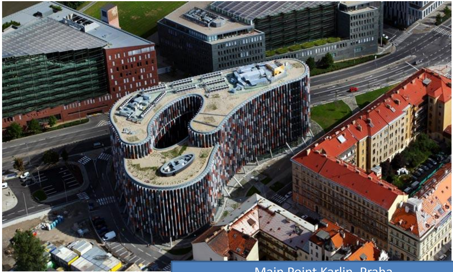
Main Point Karlin, Praha
