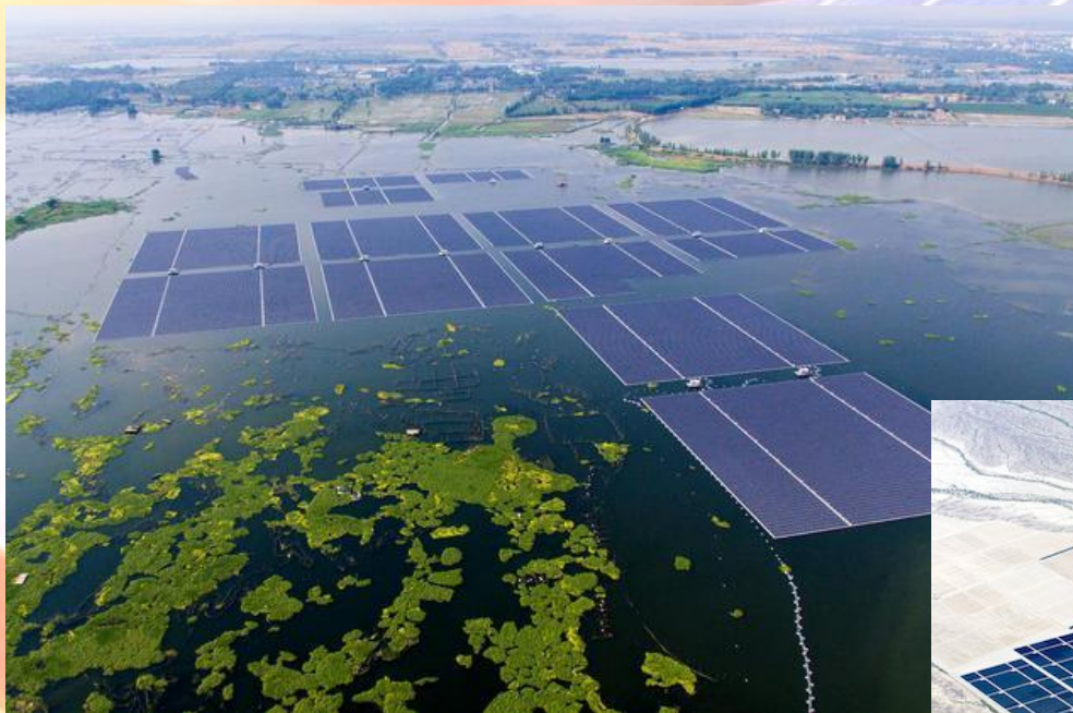
40 MW Sungrow Huainan Solar Farm
