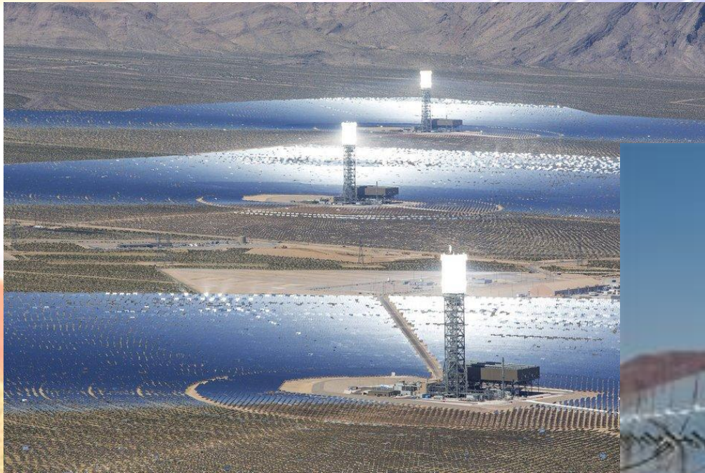
392 MW Ivanpah Solar Power Facility
