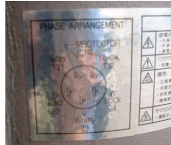
**Pay an utmost attention not to wire incorrectly for the compressor. Otherwise, the compressor may turn in reverse direction causing burn out.**
