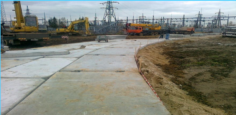
7. Concrete plates for infield roads.
