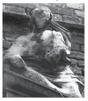
Sandstone figure over the portal of a castle, built in 1702, in Westphalia, Germany, photographed in 1908 (left) and in 1968 (right). The erosion of the figure is due to a combination of acid deposition and air pollution produced from the industrialized Ruhr region of Germany. Courtesy Herr Schmidt-Thomsen.
