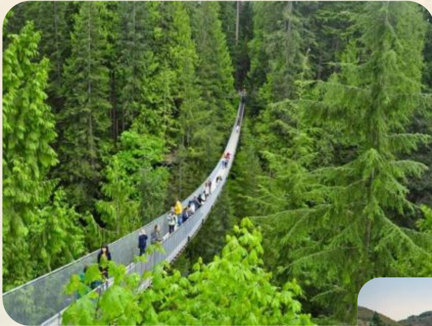
Capilano Suspension Bridge
