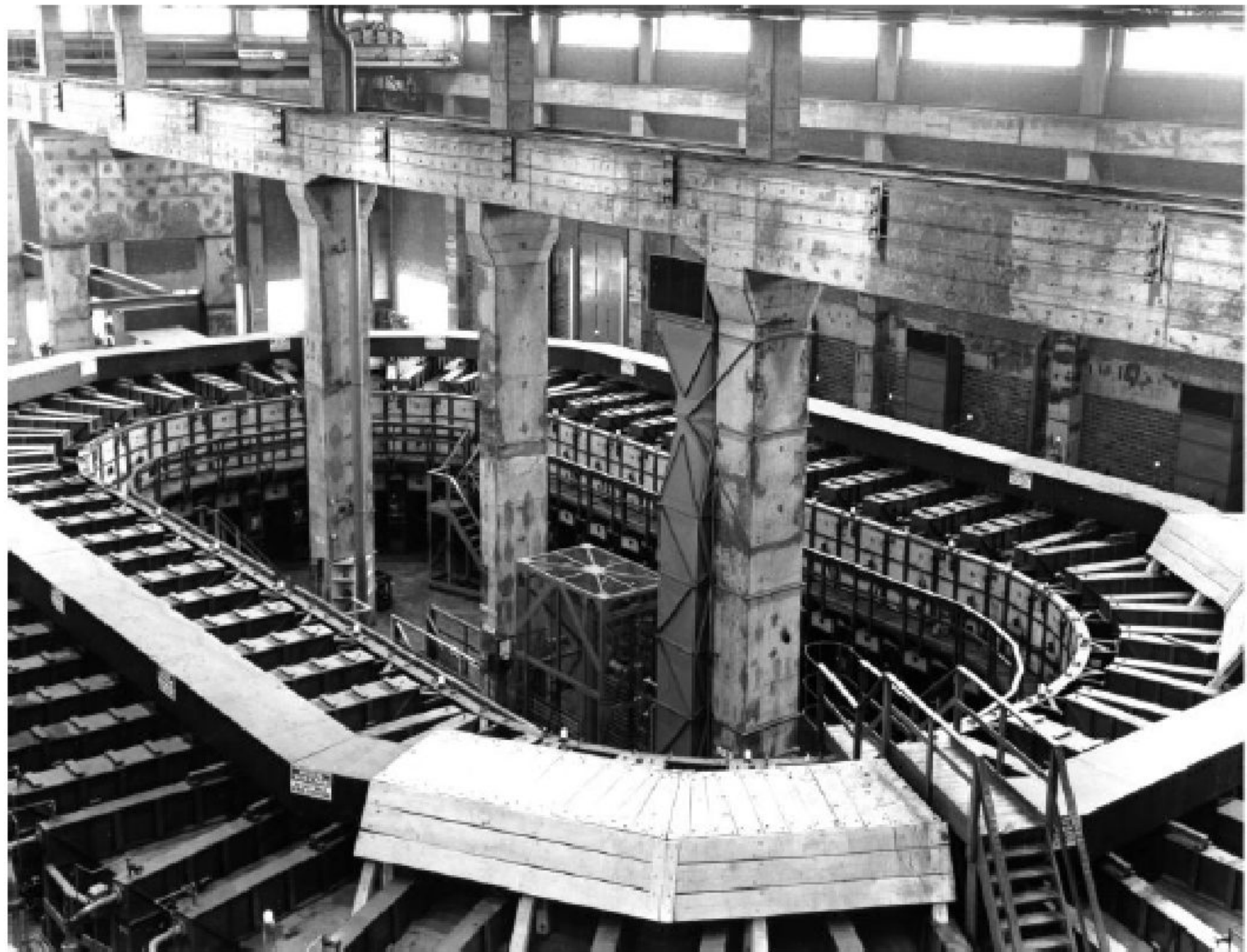
Alpha Track Calutron at the Y-12 Plant at Oak Ridge, Tennessee from the Manhattan Project, used for uranium enrichment.
