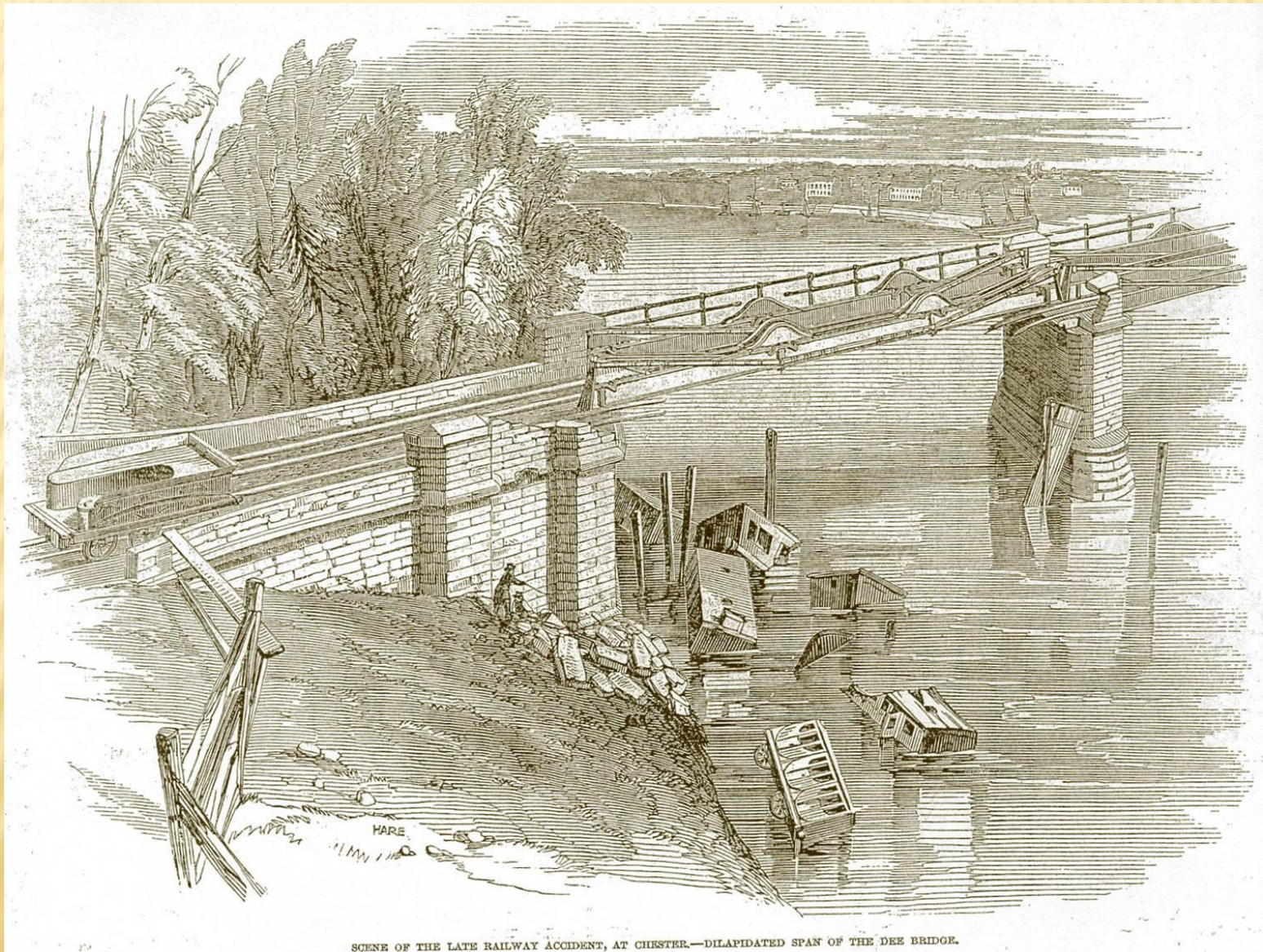
SCENE OF THE LATE RAILWAY ACCIDENT, AT CHESTER.—DILAPIDATED SPAN OF THE DEE BRIDGE.
