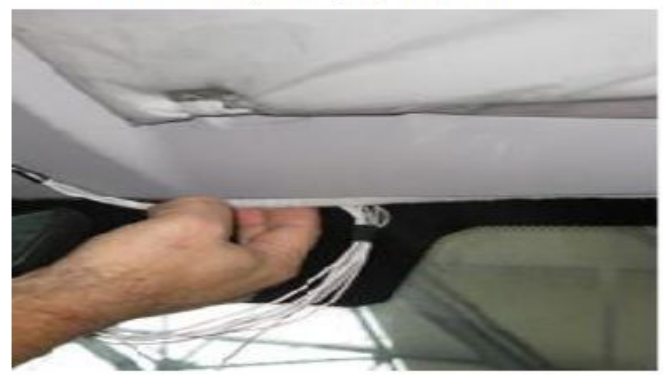
Foreseen a pvc taping for cables
