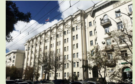
Complex of line buildings of the now
