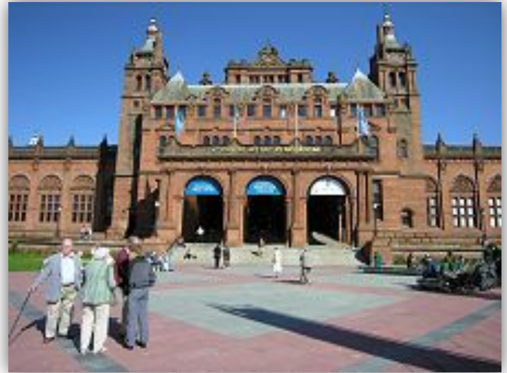
Argyle Street Entrance
