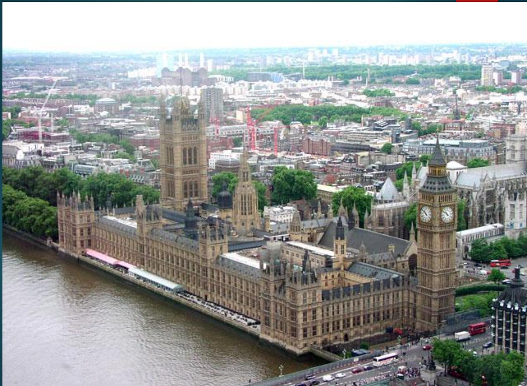
the tower leans slightly to the north-west, by roughly 230 millimetres (9.1 in) over 55 m height, giving an inclination of approximately  $1/240$ . This includes a planned maximum of 22 mm increased tilt due to tunnelling for the Jubilee line extension.[13] Due to thermal effects it oscillates annually by a few millimetres east and west.
