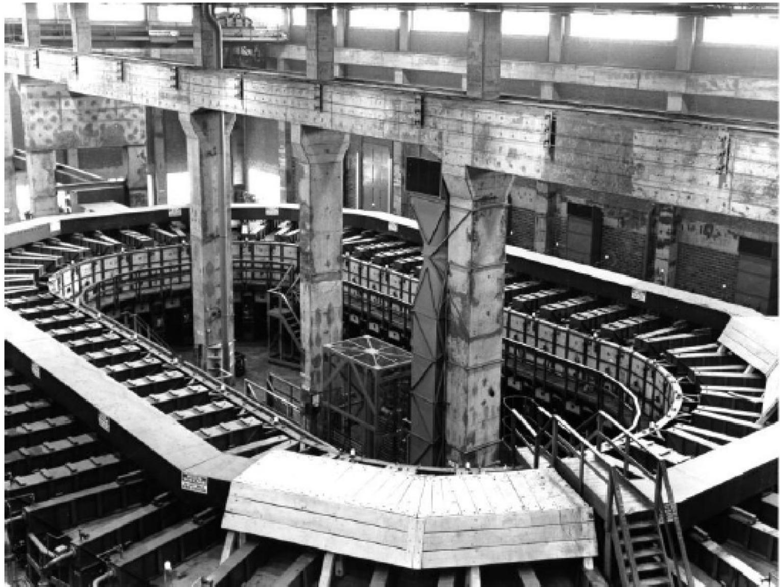
**Alpha Track Calutron at the Y-12 Plant at Oak Ridge, Tennessee from the Manhattan Project, used for uranium enrichment.**
