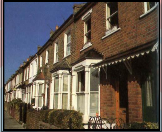
A terraced house
