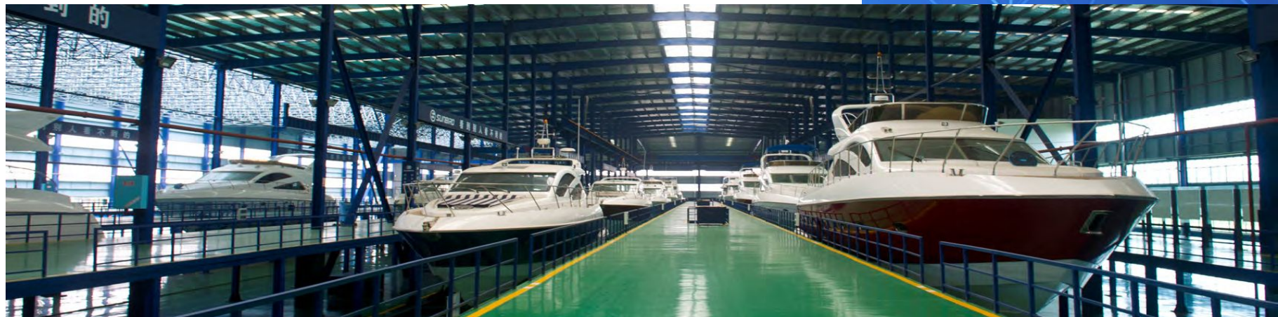
Hunan yacht modular Construction of assembly line workshop
