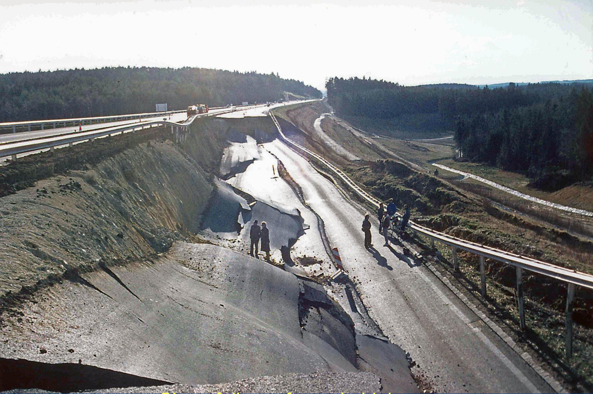
Slope failure of a main highway (1 week before Christmas)
