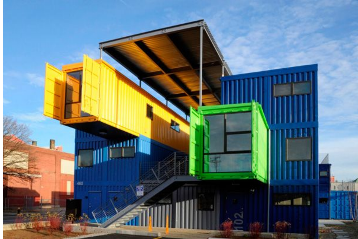
Box Office Shipping Container,
