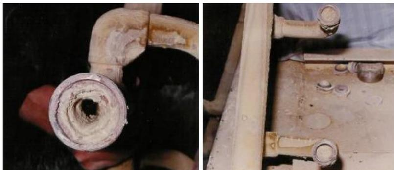
Without MHD magnetic treatment: Heavy scaling in spray rings and blockages in nozzles.
