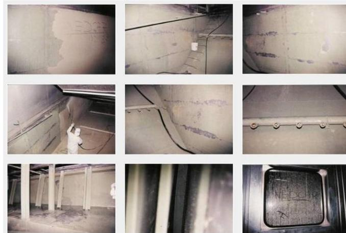
Trail period 6 months: Soft sludge and light scaling of pipe work and nozzles. Green precipitate on tank walls is slowly decreasing starting from the weld seams. NEDCAR decided to postpone the sulphuric acid rinse and permanently install the MHD magnetic modules.
