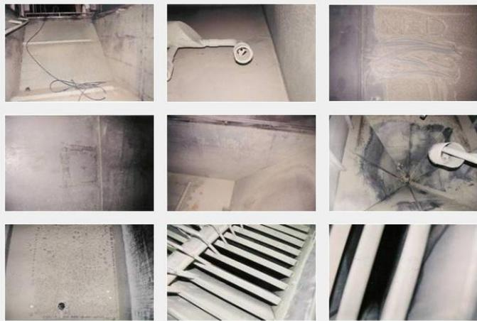
Trail period 3 months: Soft sludge can easily be sprayed off, acid rinse of heat exchanger after 3 months.
