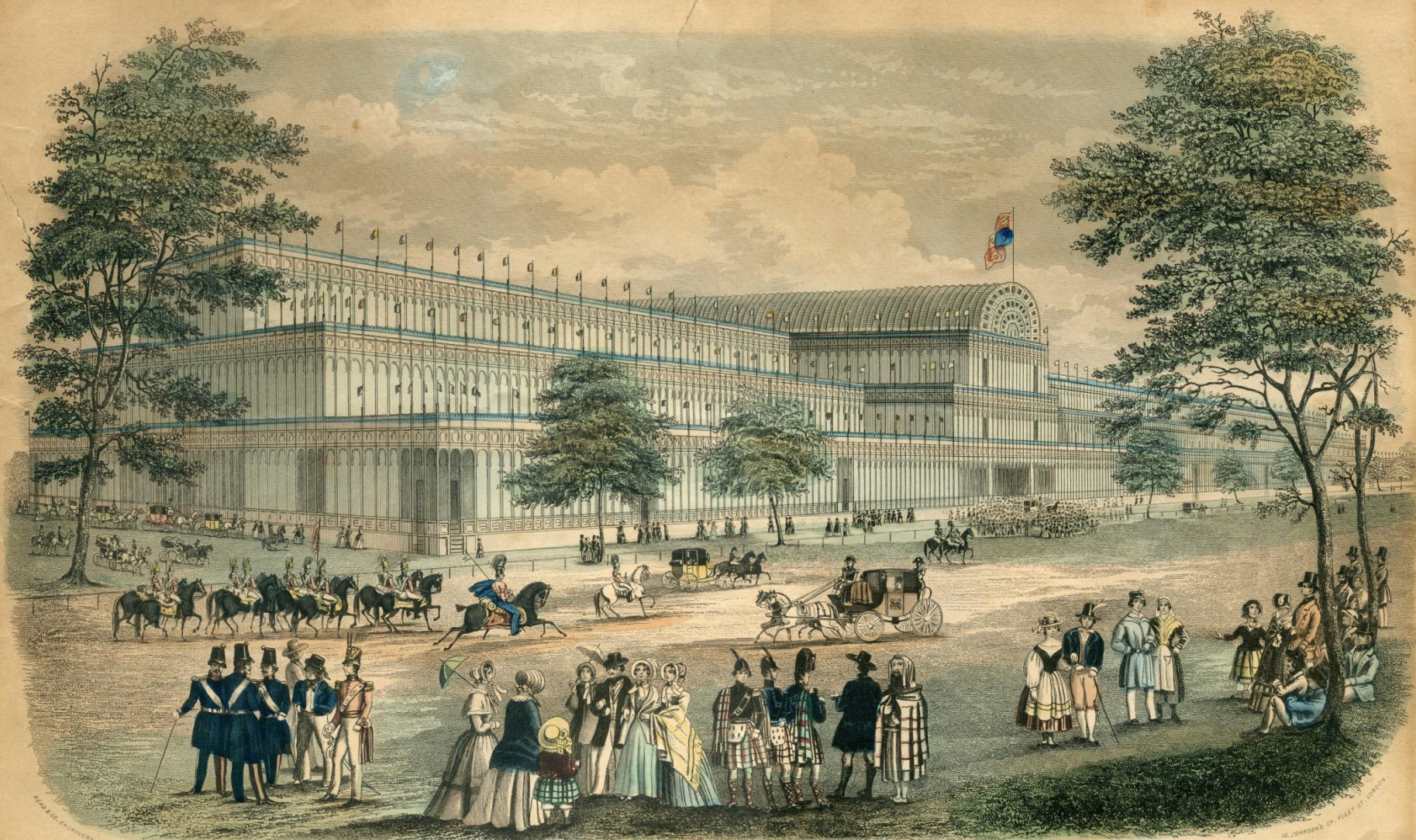
VIEW FROM THE KNIGHTSBRIDGE ROAD OF THE CRYSTAL PALACE IN HYDE PARK FOR GRAND INTERNATIONAL EXHIBITION OF 1851. Dedicated to the Royal Commissioners.
