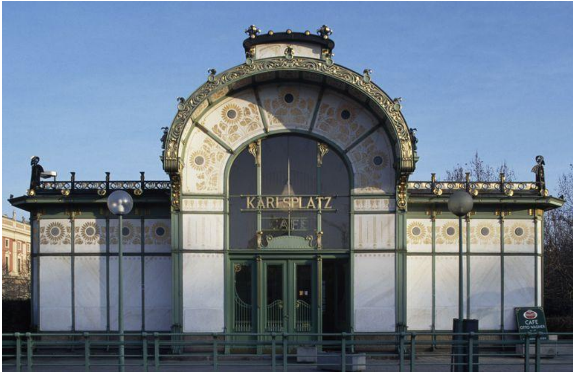
Railway station Karlsplatz Stadtbahn, Otto Wagner
