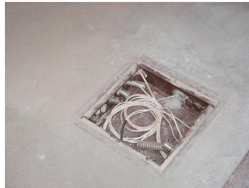
Wells with cables in the concrete floor.
