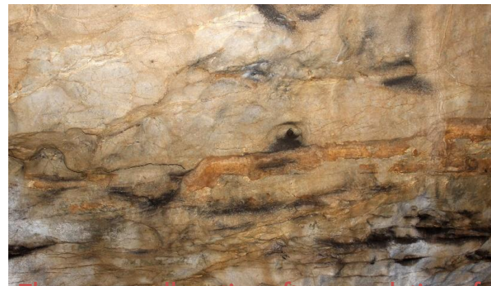
The same wall section after completion of works
